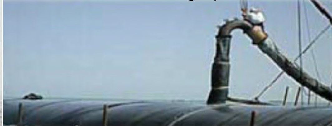
Geotube Filling Operation
